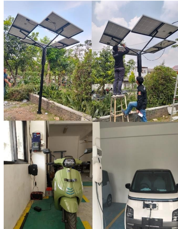
Figure 3. Schematic of solar photovoltaic trees for an electric vehicle charger
